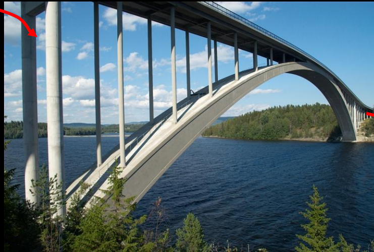
The Sandö bridge, reinforced concrete , world's largest span for a concrete bridge when it was constructed in 1943 (span: 264 m)
