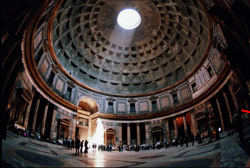
The Pantheon, unreinforced concrete (Dome structure, diameter: 43 m)
