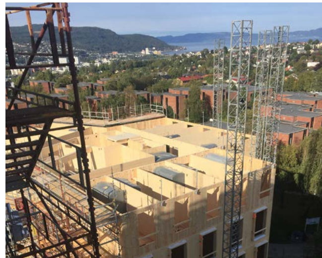
Example with no weather protection, Moholt 5050, Trondheim, Norway.
