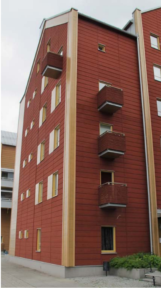
Balconies made of CLT, Inre Hamnen, Sundsvall, Sweden.
