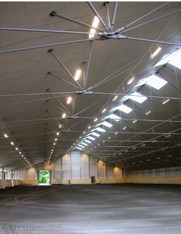
Trussed CLT roof, Flyinge Riding School, Lund, Sweden.
