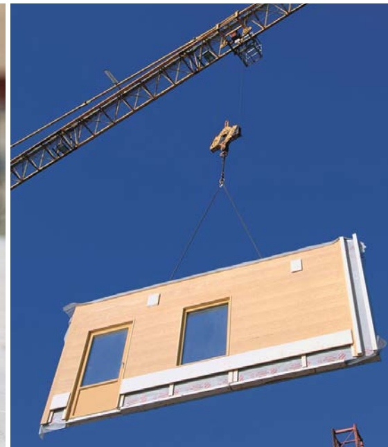
Lifting a prefabricated wall unit.
