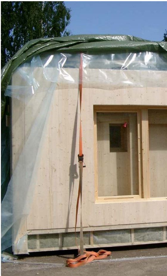
Prefabricated wall units being unwrapped for assembly.
