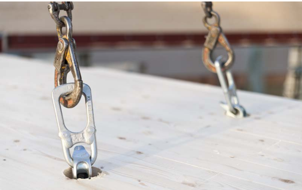
Spherical head lifting anchors fixed with wood screws.
