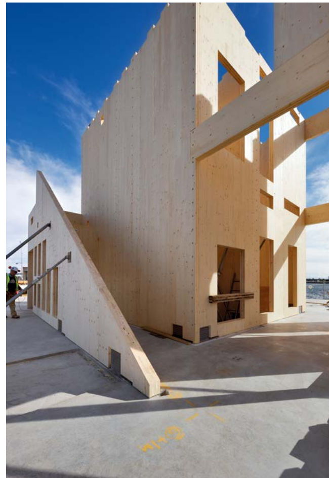
Assembly of CLT walls.
