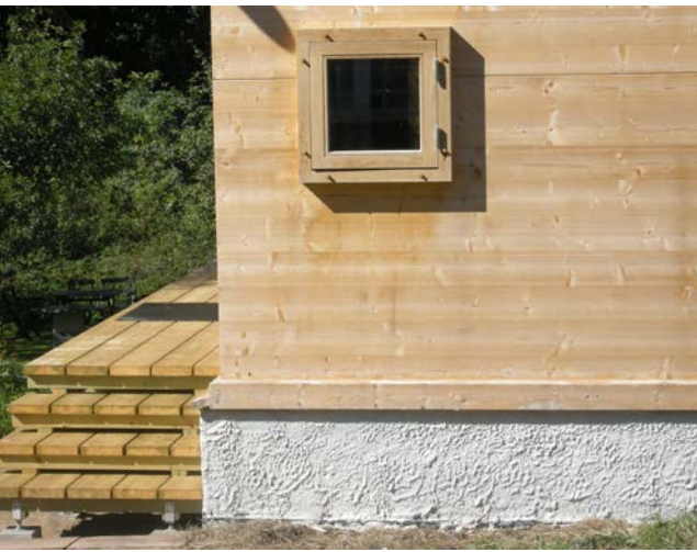
Summer house under construction, Öland, Sweden.
