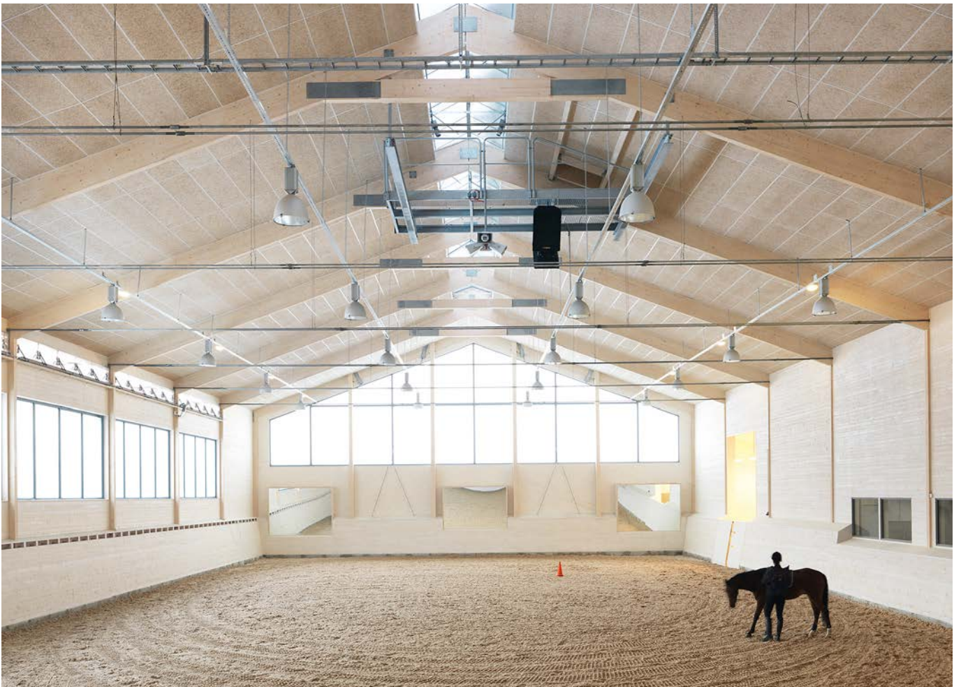
Indoor riding arena with walls and boards in CLT, Sätra, Sweden.
