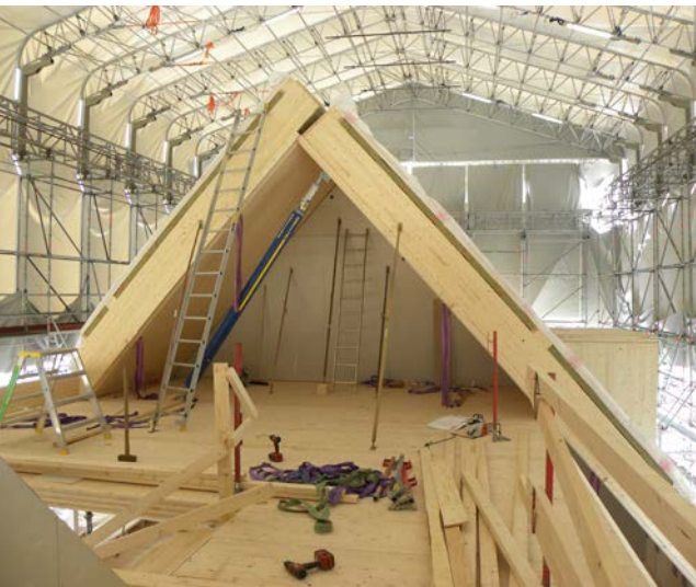
Assembly roof, Sundbyberg, Sweden.
