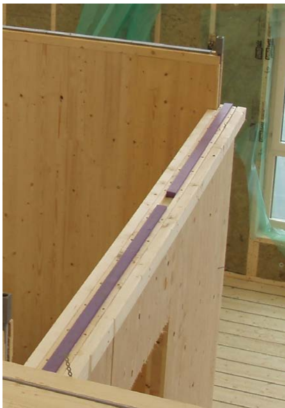
Example of a vibration-damping intermediate layer.
