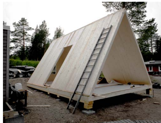
Assembly of a summer house, Skellefteå, Sweden.
