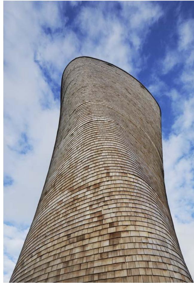
Ventilation tower with CLT frame, Stockholm, Sweden.
