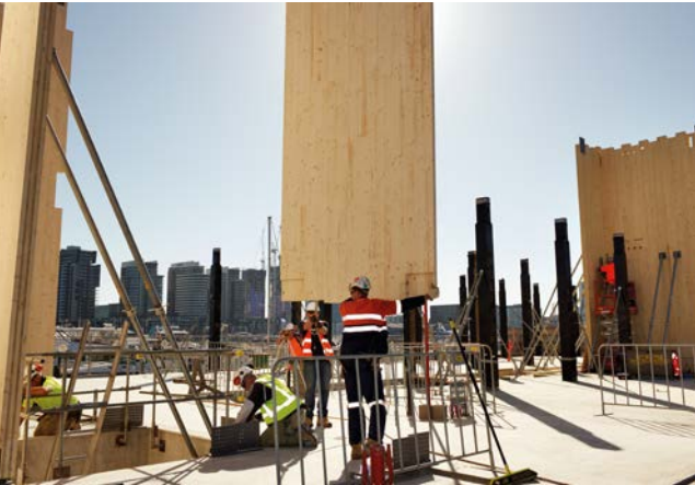
Assembly of CLT-walls.
