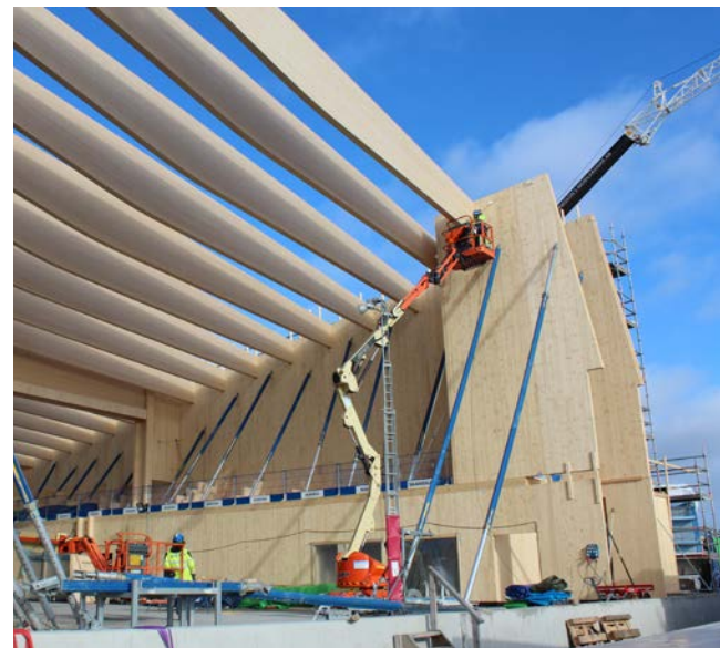
Stabilising using braces during construction.
