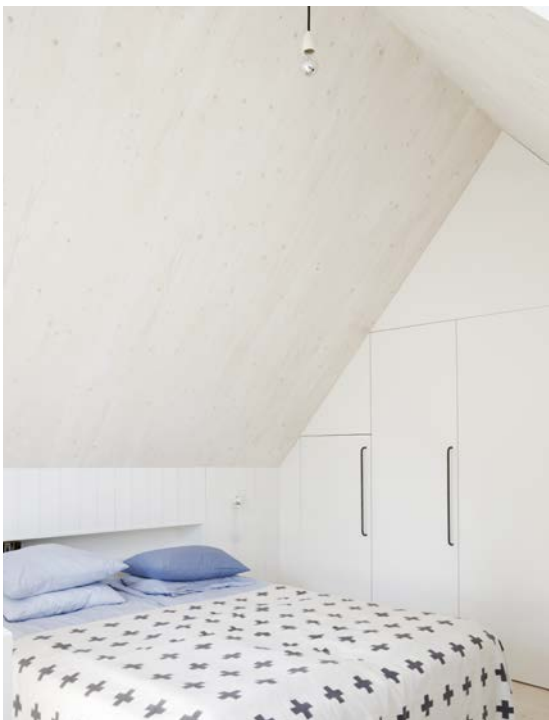
Example of a roof structure with load-bearing and stabilising CLT panels, which also contribute to a good indoor climate.
