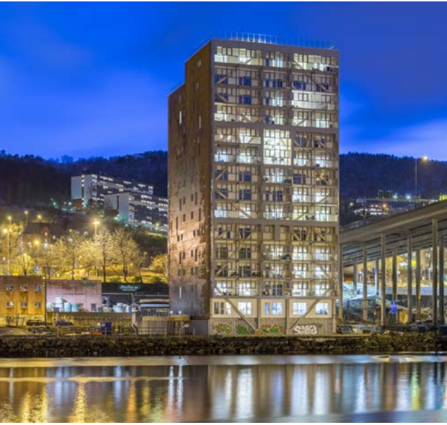
Multi-storey building, Bergen, Norway.
