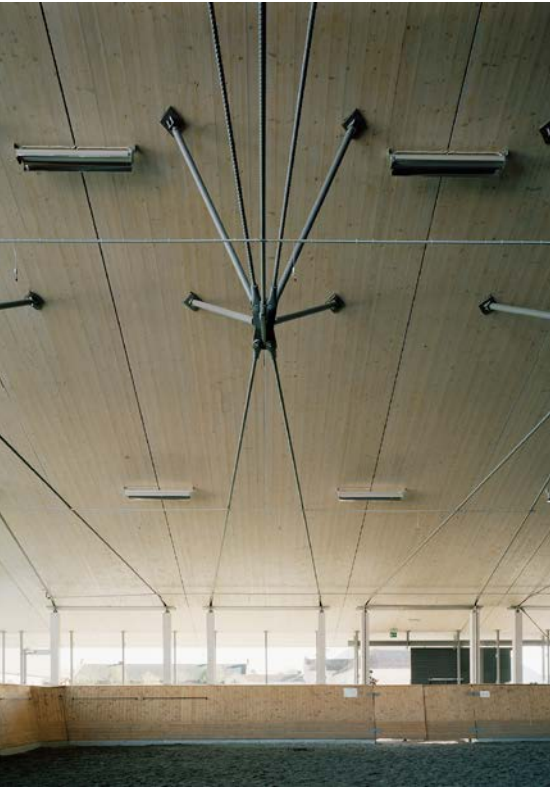
Supported roof of CLT, Flyinge, Lund, Sweden.
