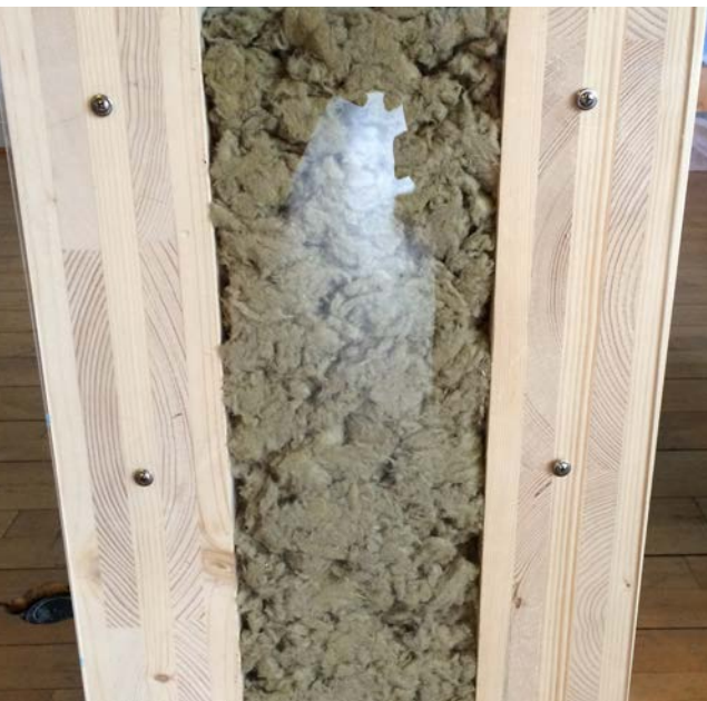
Example of partitional wall.
