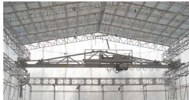
Tent with crane.
