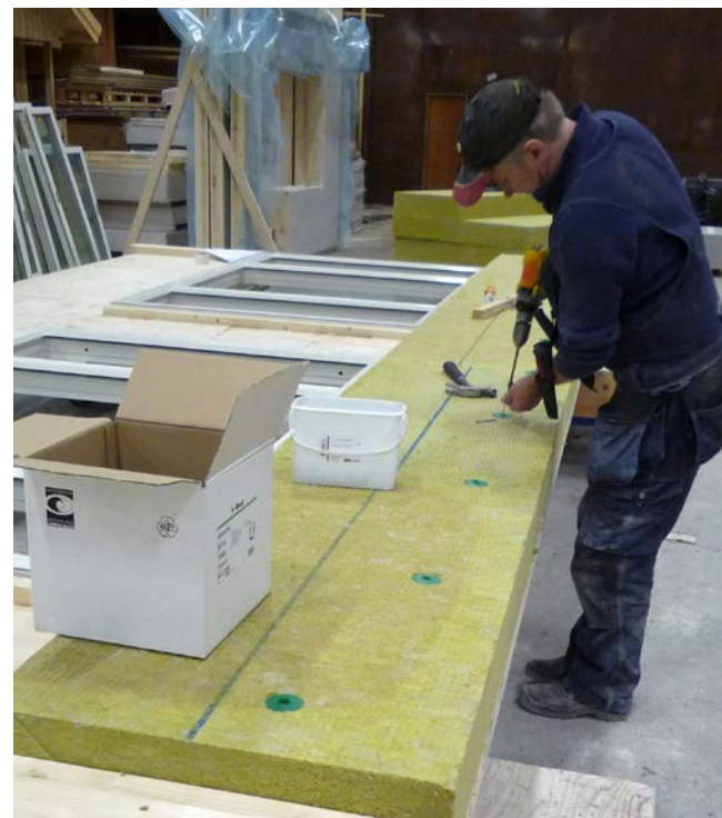
Insulation of CLT wall.
