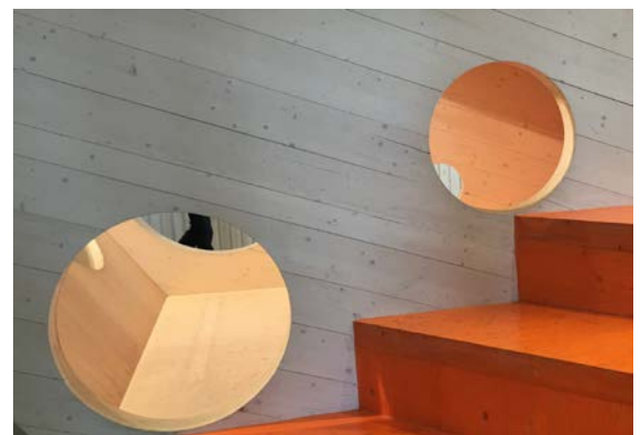
Example of holes cut in CLT. The structure of the panels provides wide scope for architectural design flourishes and adaptation to the client's wishes and requirements.
