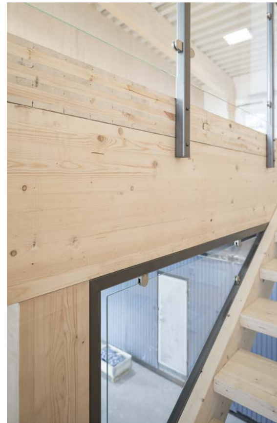
Floor made of CLT, Ålta, Sweden.
